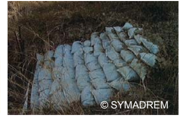
Upstream slope sliding during flood draw down
