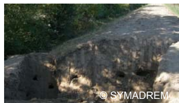
In a former badger burrow partially plugged, not visible and unknown, after hydraulic fracturing
