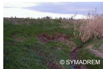
Downstream slope sliding during flood
