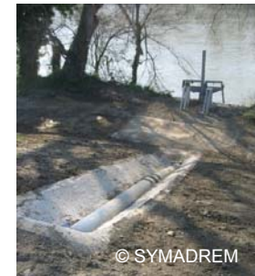
350 crossing hydraulic structures
