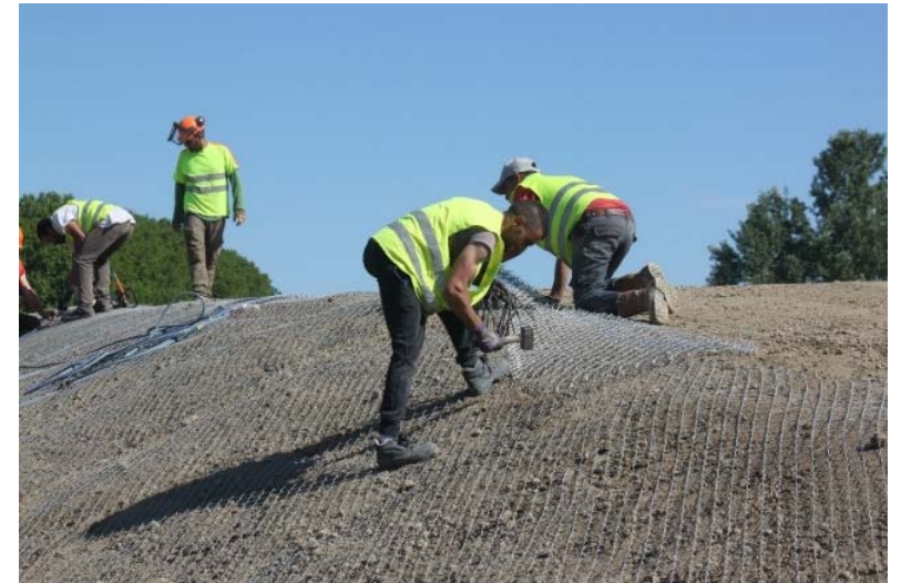
New levee with grid against burrowing Probability = 0,001
