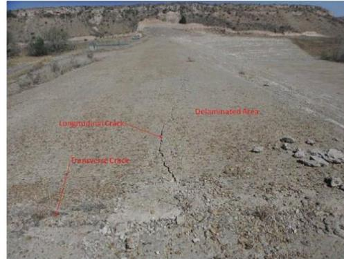
13. Transverse crack (foreground) in dam crest at STA 6+50 in foreground, looking left. Longitudinal crack extends from transverse crack about 20 feet to left. Top lift is unbonded left of transverse crack and downstream of longitudinal crack.
