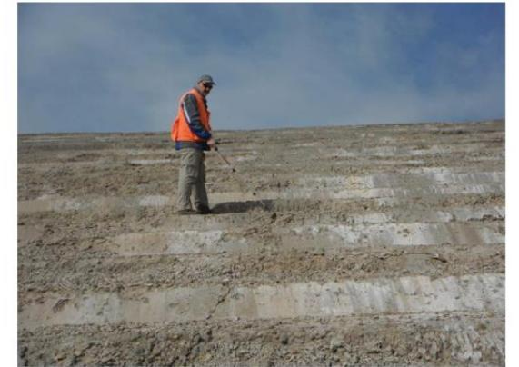
16. Downstream slope near STA 6+50, looking upstream. Note typical transverse crack.
