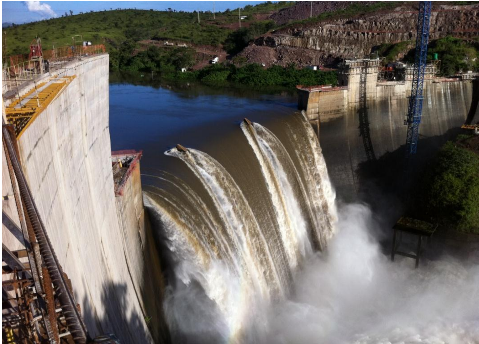
Manso/ Overflow resistance of concrete dams
