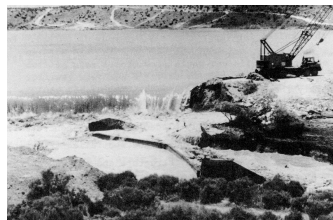
Spillway Breach
