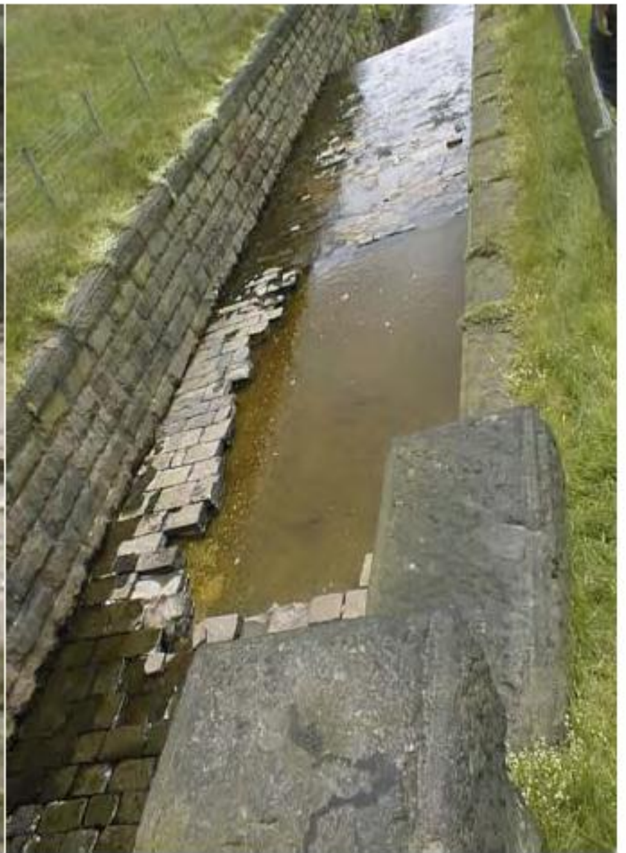
Figure 2.17 Examples of invert failures of stepped masonry spillways
