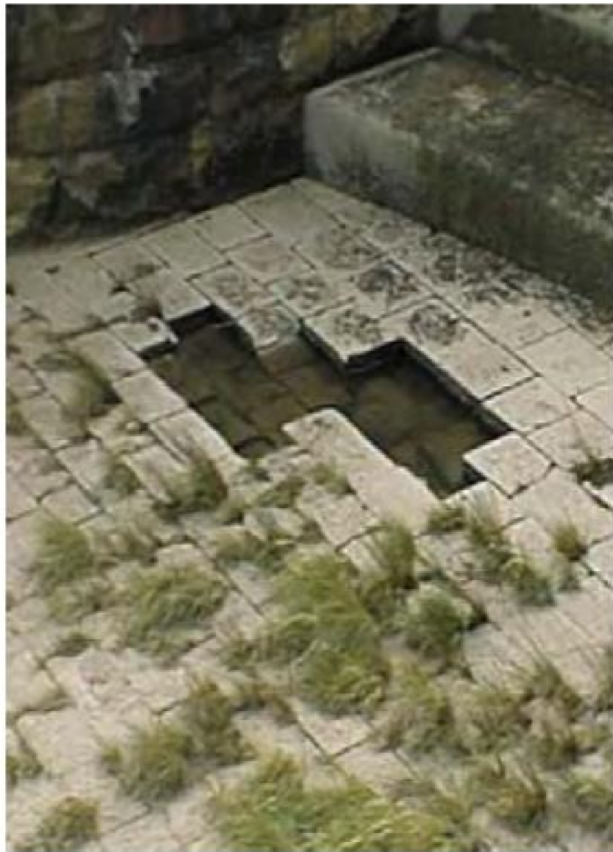
Figure 2.17 Examples of invert failures of stepped masonry spillways
