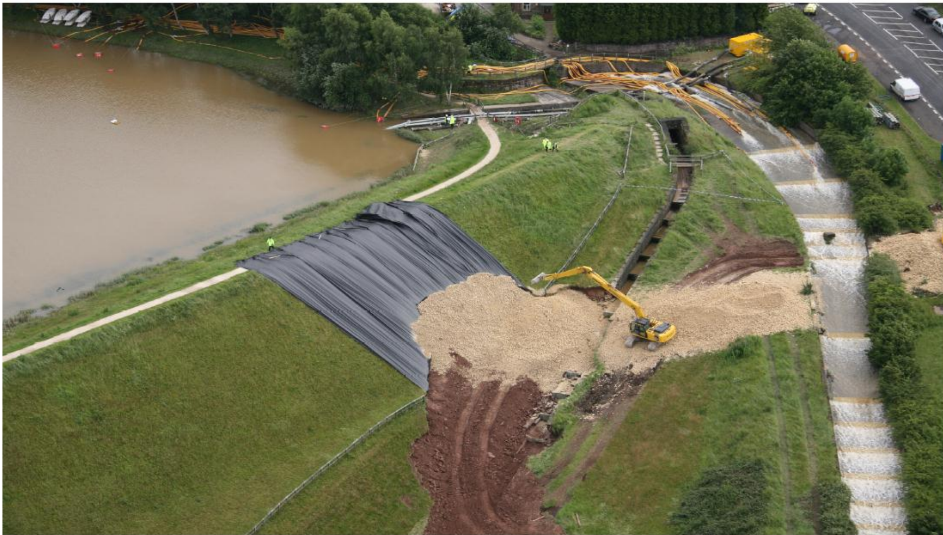
Figure 1 - Works in progress filling scour hole
