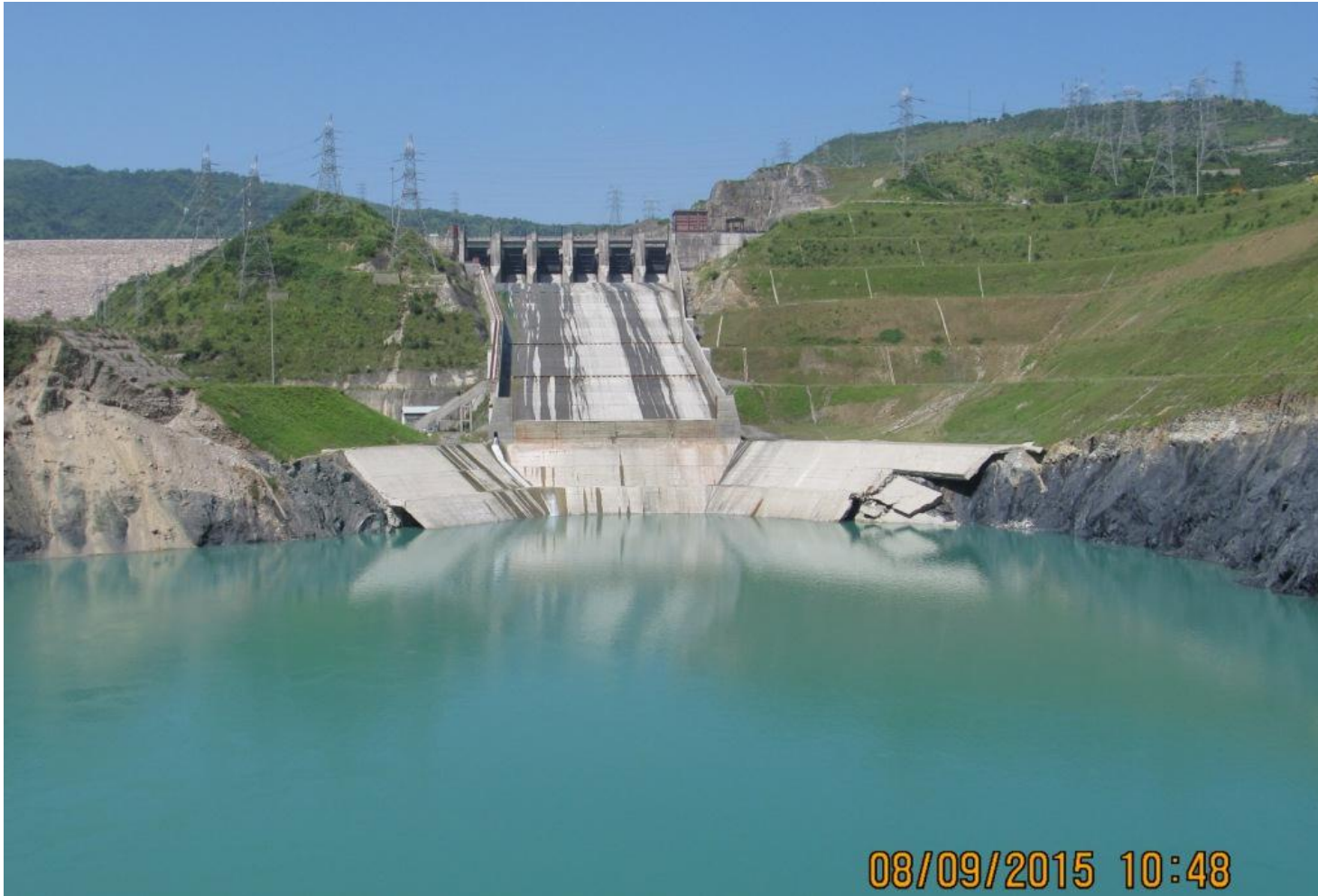
Re-circulating flow downstream
