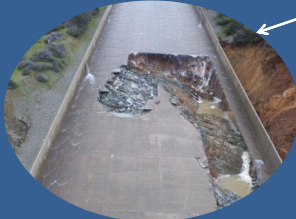
Additional SS Damage
