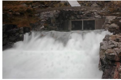
Step 5, Overtopping 1,5 m
