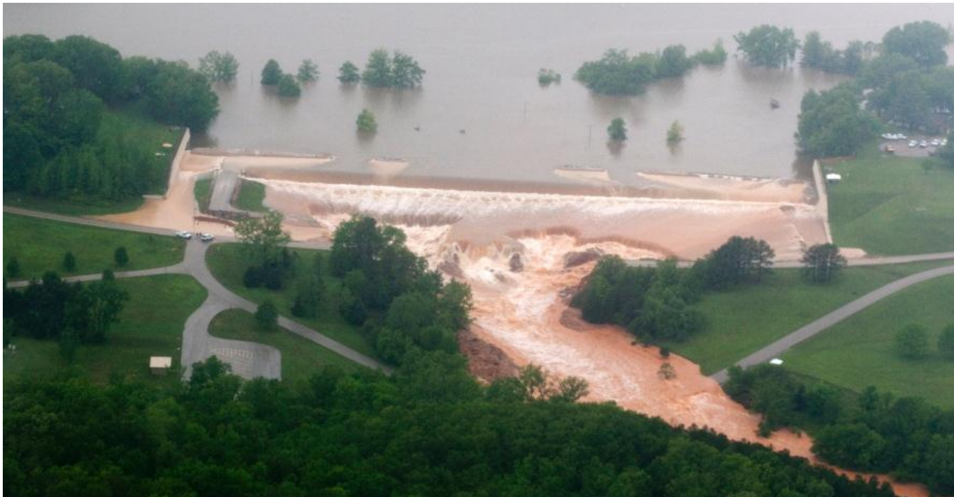
Prototyp of an erodible barrier for a controlled flooding of a polder US Corps of Engineers
