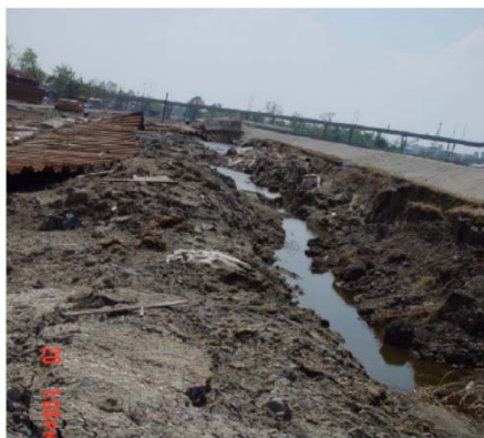
Initial Stage A: Erosion due to overtopping on the Citrus Back Levee
