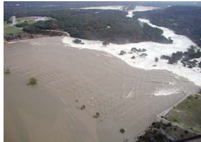
USACE Canyon Dam Spillway
