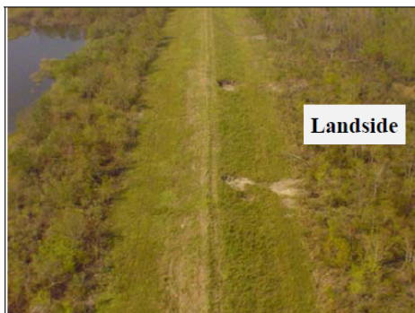
Initial Stage A: Erosion due to overtopping on the Citrus Back Levee
