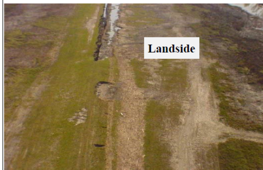
Stage C: Crown scour along the MRGO levee in St. Bernard Parish
