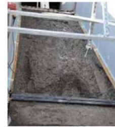
a. Bare clay soil slope, upper 20 ft
