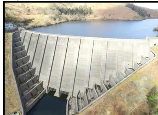
Clywedog Reservoir (Severn Trent)
