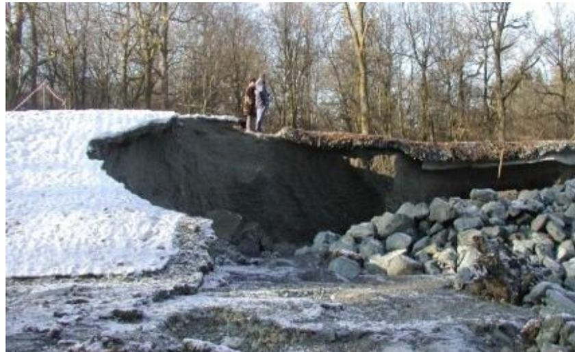
Erosion / Stability of hydraulic structures
