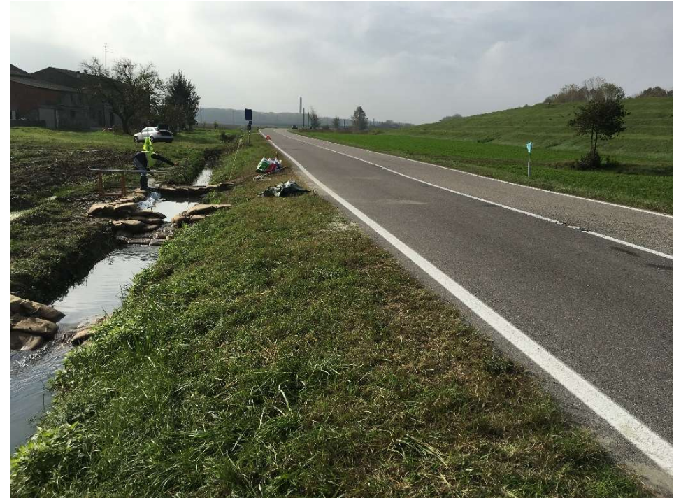
Picture of the sand boil in equilibrium condition, after sandbagging
